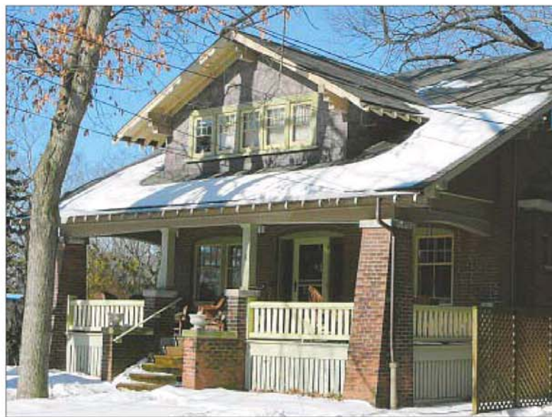
Toronto's Craftsman bungalows feature low-pitched gabled roofs with deep eave overhangs, decoratively shaped rafter tails and exposed roof beams.
