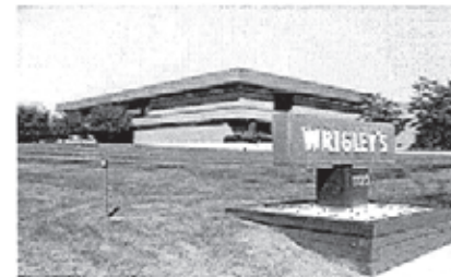
The Wrigley Building by Gordon Adamson on Leslie Street.
