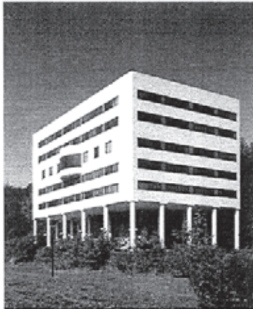
The Administration offices of the Lipa Green Building, soar above the valley on 3-storey pilotis. Photographer unknown, courtesy of J. Markson.
