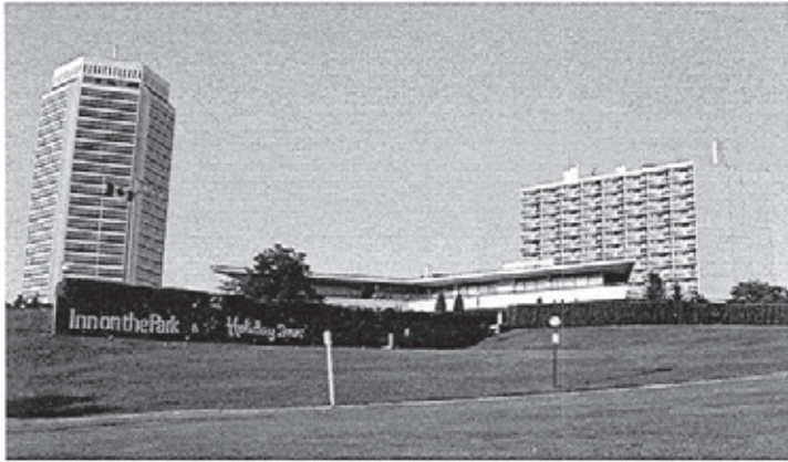
In a view from Eglinton Avenue, the projecting forms of the Inn on the Park appear to soar over the site.
