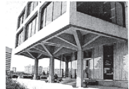
Expressive columns support three sides of the building with their tree-like forms.
