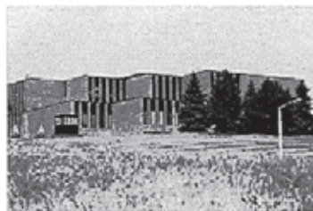
The IBM Offices on Don Mills designed by N.O.R.R.
