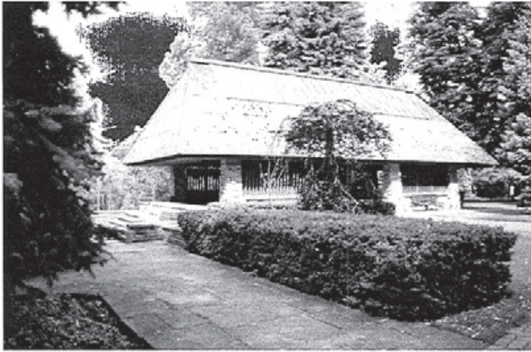
The Civic Garden Centre Pavilion, a shelter in Edwards Gardens is reminiscent of the German architect, Gunnar Asplund's Woodland Chapel.
