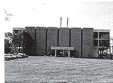
The south facing front elevation with its projecting bays, house the building services.
