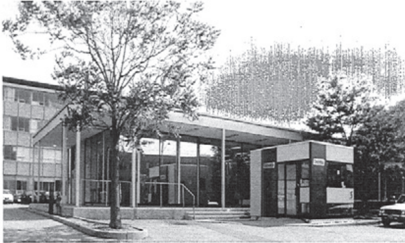
The Bank of Nova Scotia and the adjacent Bank of Montreal are both glazed entirely with only the vaults as solid elements.
